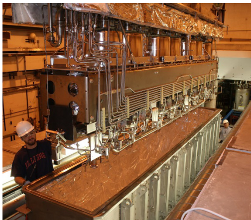
Figure 4: Cold mass assembly loading into the cryostat vacuum vessel in the tunnel.
