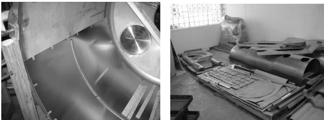
FIGURE 6. Example of magnetic shield installed on the inside surface of a vacuum vessel using batten strips (left). Aluminum thermal shield parts ready for assembly (right).
